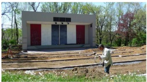
Scott Balsbaugh, an electrician for Woodland Contractors, pulls wire through a conduit buried underneath the new terraces at Veterans Memorial Amphitheater in Coleman Memorial Park. The wires will be connected to light stanchions that were removed to allow the asphalt to be removed and the hillside terraced. (John Latimer / Lebanon Daily News)
